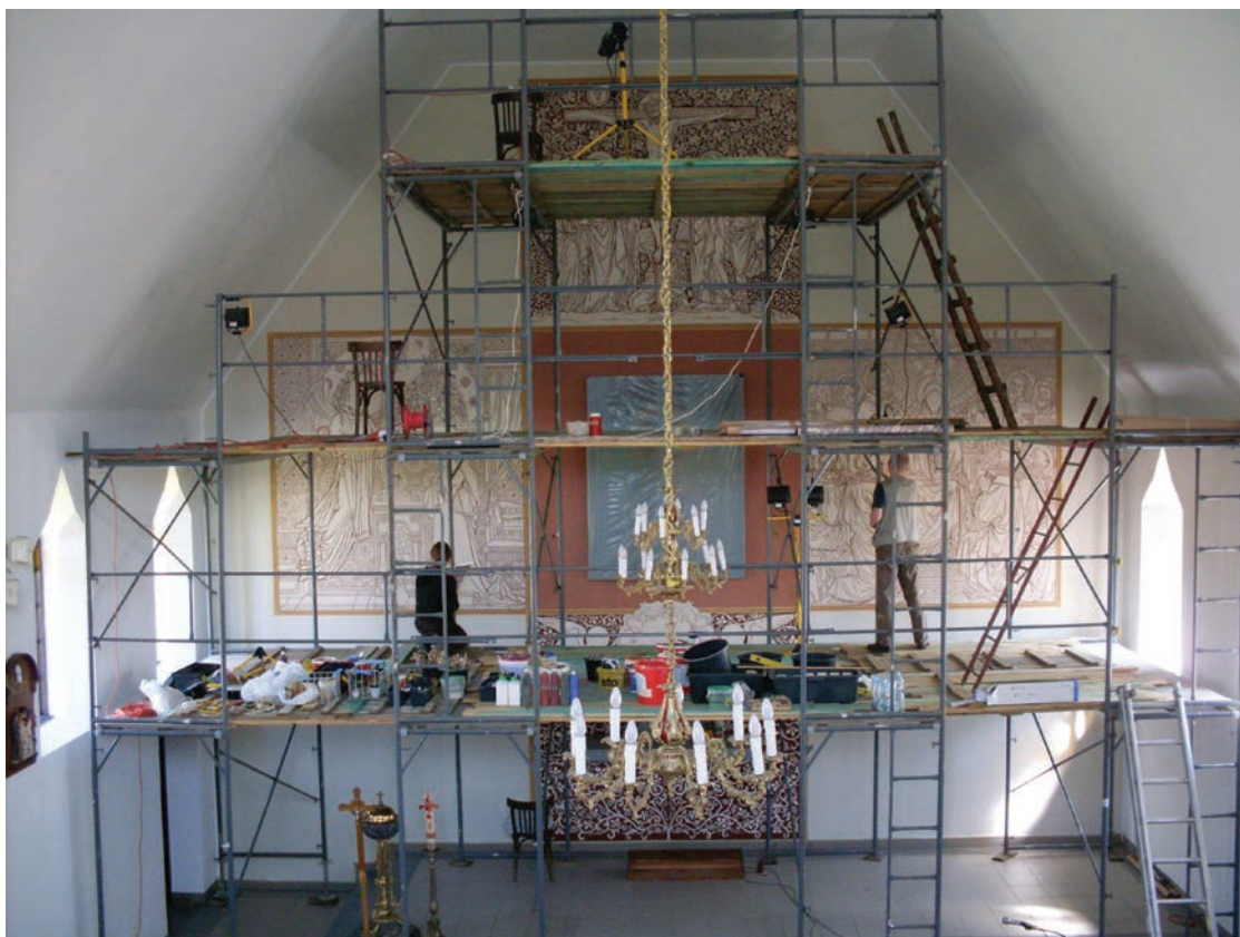
Ściana oltarzowa w trakcie prac / The altar wall during works
